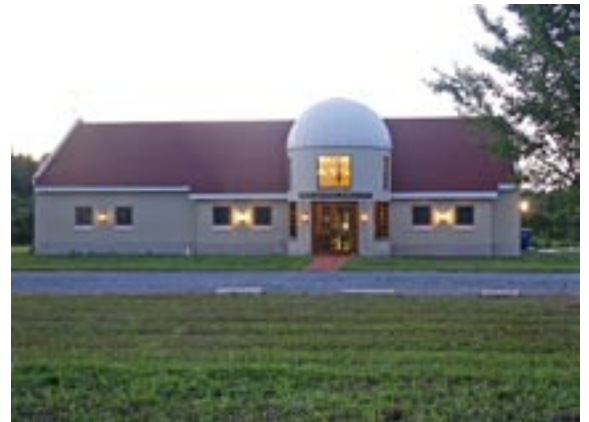
The new Deep Landing Workshop
